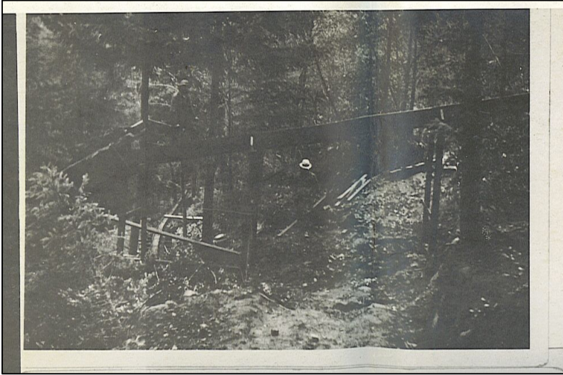
Fig. 12. C.S. Cooke inspecting an elevated section of sluice (Reproduced from F.E. Cooke, private collection, circa 1934).
