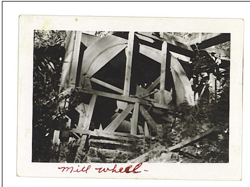
Fig. 7. 16 foot water wheel drove sawmill, ball mill, and generator (Reproduced from F.E. Cooke, private collection, circa 1934).
